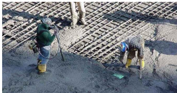
Gambar 4.18 In-Situ Concrete for Floor Slabs
