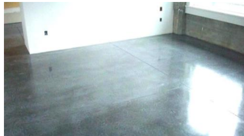
Gambar 4.25 Finished Concrete for Flooring
