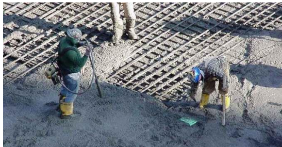
Gambar 4.19 In-Situ Concrete for Roof Construction
