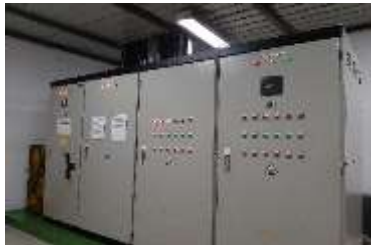
Mesin pengatur suhu cold storage
