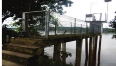
FIGURE 7. Sanggau Telemetry Station, Field Documentation on March 14, 2015
