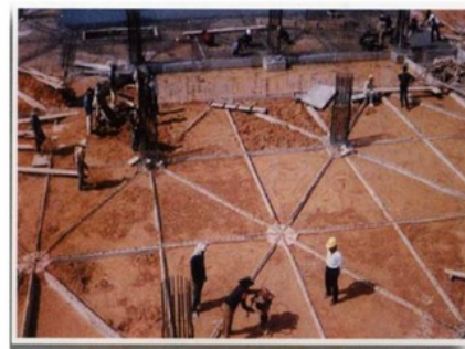
(b) The compaction of filled soil
