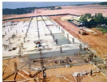
(c) The raft plate construction
