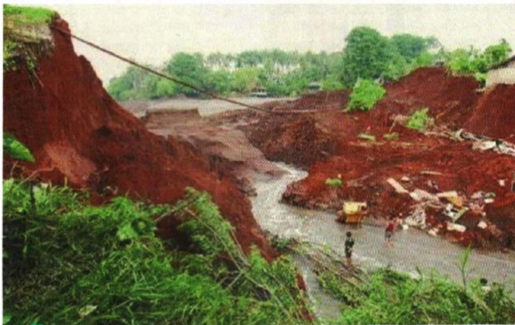
4 Fig. 4.12 Collapse of the Situ Gintung dam on March 27, 2009
