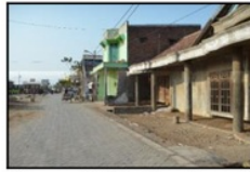
Figure 3. The Road condition as the main access in Tambak Lorok
