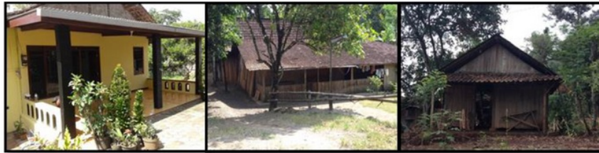
Figure 5. Building Construction of East Ungaran District (Analysis, 2015)
