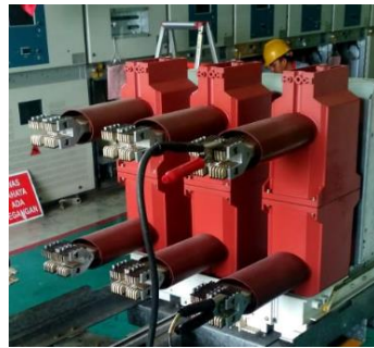
Gambar 2. 13 PMT 20 KV
