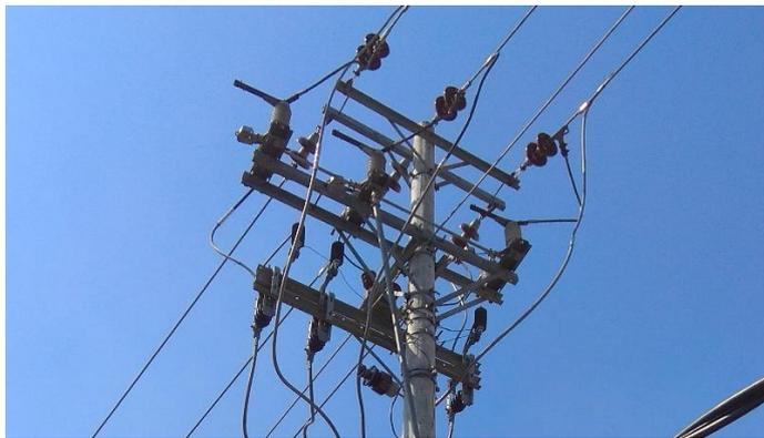
**Gambar 2.8** *Air Break Switch* (ABSW)
