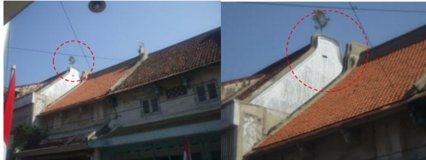
Figure 10 Typical Konde Roof
