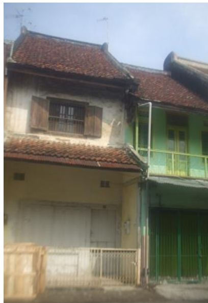
Figure 3 The Traditional Housing Facades in Semarang Chinatown
