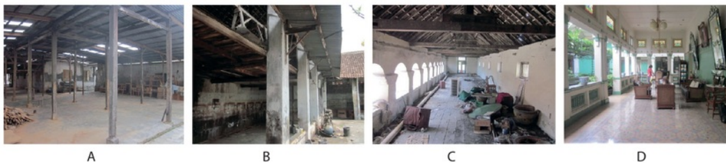
Fig. 6. Posts, beams, and arches: A and B. the factory of Harjodikoro houses I; C. the upper stair of loteng in the Cokrosumarto's house II; D. the back veranda of the Cokrosumarto houses I Source: the Authors.
