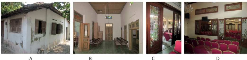
Fig. 7. Walls and openings. A. The old house in Laweyan; B. The Harjodikoro's house I (1900s); C and D. The Cokrosumarto's house II (1950s): The openings connecting rooms in the main house that are comfortable for wedding party Source: the Authors.
