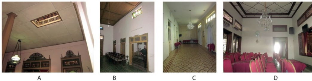
Fig. 8. Ceilings, sky lights and ventilation holes. The Harjodikoro's house I: A. The dalem ; and B. The pringgitan . The Cokrosumarto's house II: C. The toko ; and D. The gandok of the main house Source: the Authors.
