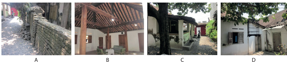
Fig. 4. The ancient house is preserved at the old Kampung of Laweyan: A. The old brick construction; B. The incorporation of brickwalls with wooden structures; C.The brick pillars; and D.The exterior of the wall house
