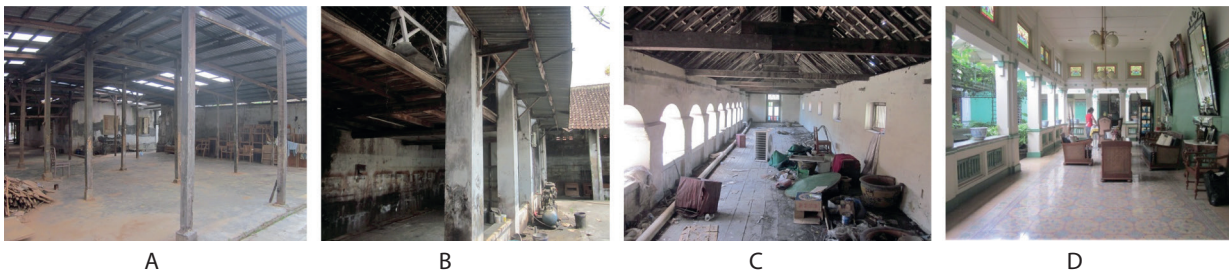
Fig. 6. Posts, beams, and arches: A and B. the factory of Harjodikoro houses I; C. the upper stair of loteng in the Cokrosumarto's houses II; D. the back veranda of the Cokrosumarto houses I Source: the Authors.
