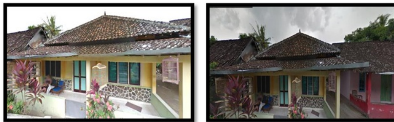
Figure 2. The condition of housing in Tegaldowo village
