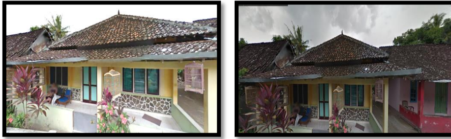
Figure 2. The condition of housing in Tegaldowo village
