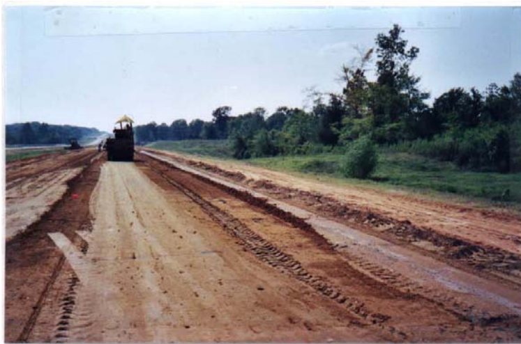
Gambar 12.b. Finish-compaction dengan Rubber-tired-roller 10
