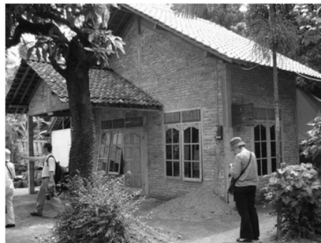
Figure 2. In-situ core house as one type of post disaster housing reconstruction program
