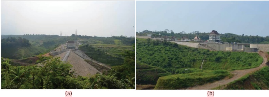
FIGURE 4. Existing Condition at Segment 3 of Jatibarang Green Belt Area.
