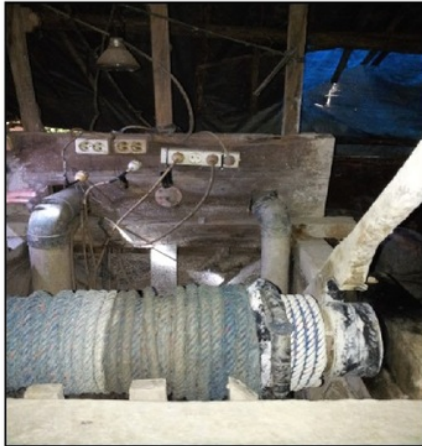
Fig. 2 Electricity and air lines to the site
