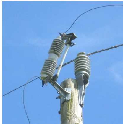
Gambar 2.7 Fuse Cut Out
