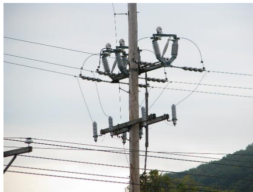
Gambar 2.11 Lightning Arrestter
