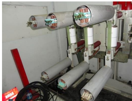
Gambar 2.8 PMT 20KV
