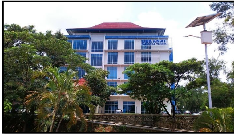
Gambar II.1. Aset Gedung Kampus UNDIP Tembalang
