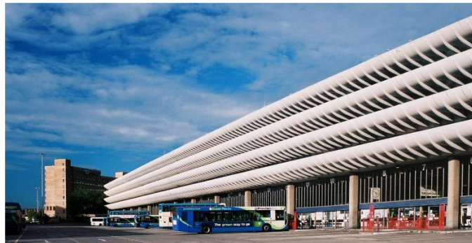
Gambar 6.5 Preston Bus Station Sumber : en.wikipedia.org, 2016
