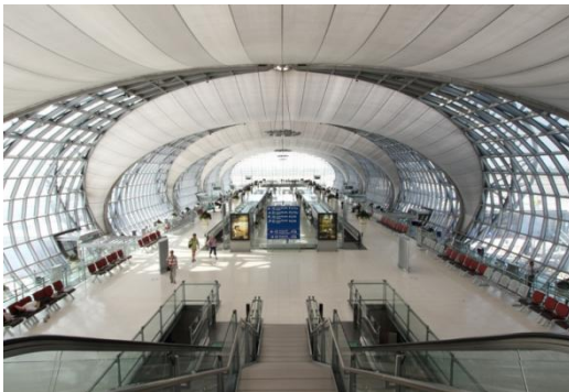
Gambar 5.14 Hall Bandara Internasional Suvarnabhumi Sumber : acrhdaily.com
