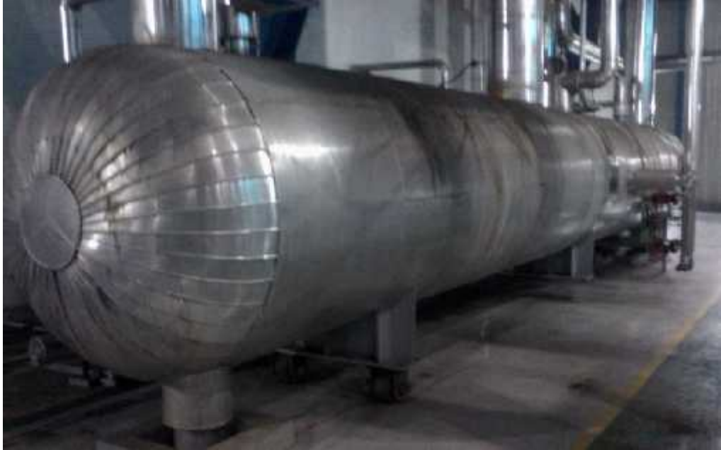
Gambar 2.11 High Pressure Heater
