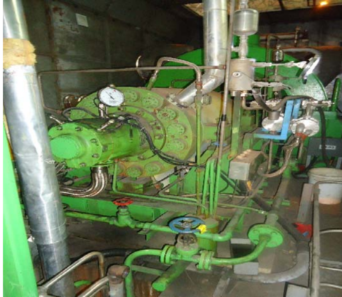
Gambar 2.5 Turbine Boiler Feed Pump
