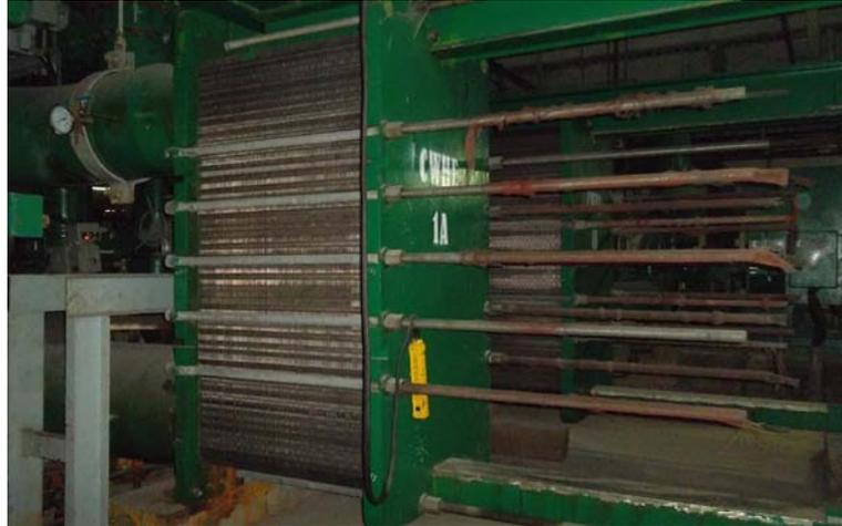
Gambar 2.17 *cooling water heat exchanger*
