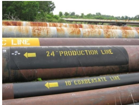
Gambar 3.47. Pipeline Production Gathering Line (PGL) 24 in di area 7 ke CGS 1.
