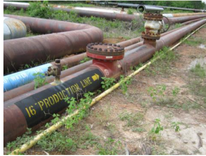
Gambar 3.46. Pipeline Production Gathering Line (PGL) 16 in di area 7 ke CGS 1.
