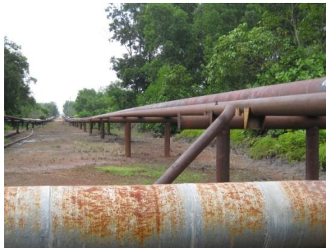
Gambar 3.48. Support pipeline Production Gathering Line di area 7 ke CGS 1.
