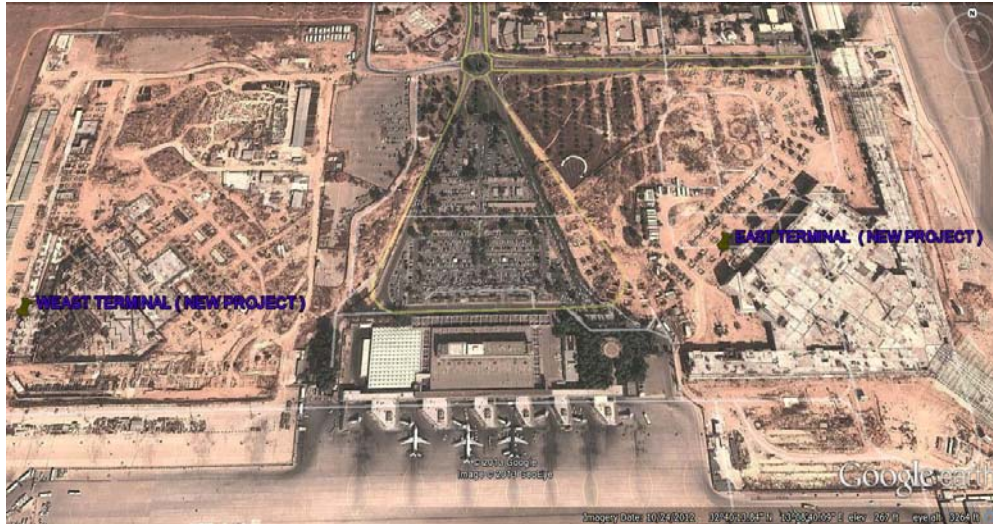
Figure 1-4 New Terminal Under Construction
