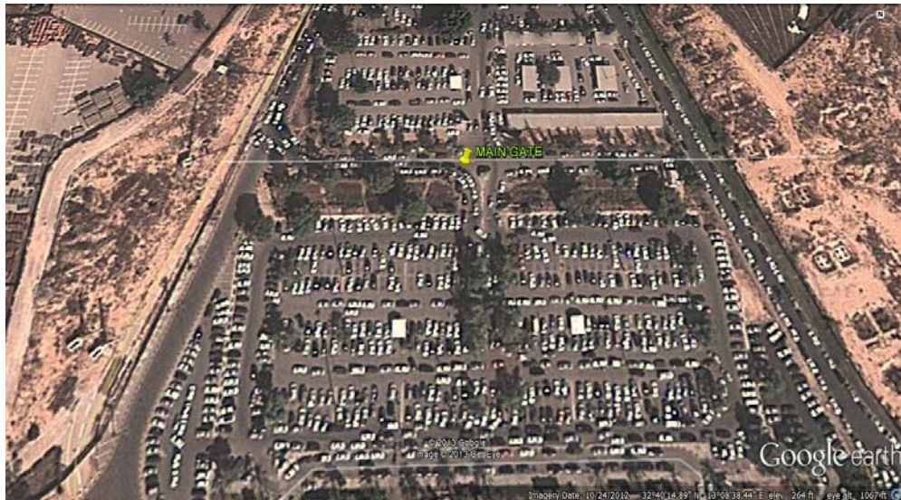
Figure 1-6 The main Gate of Tripoli International Airport
