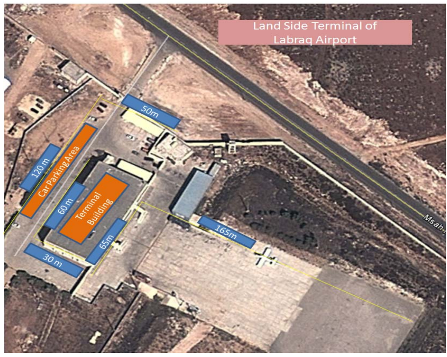
Figure 6. Terminal of Labraq Airport in Libya
