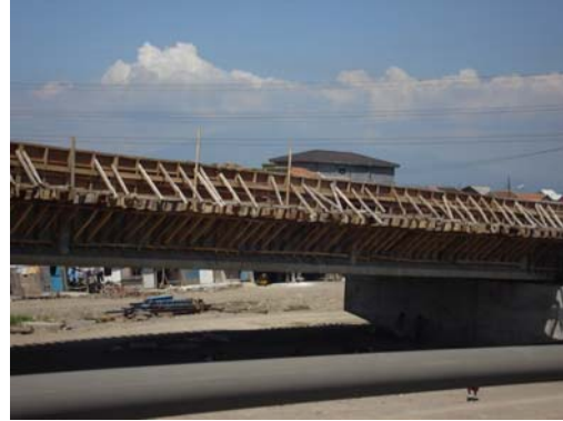
Gambar 1.2 Jembatan Kali Banjir Kanal – Banger
