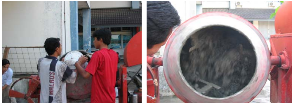
Gambar 3.6. Pencampuran material beton ( mixing beton )
