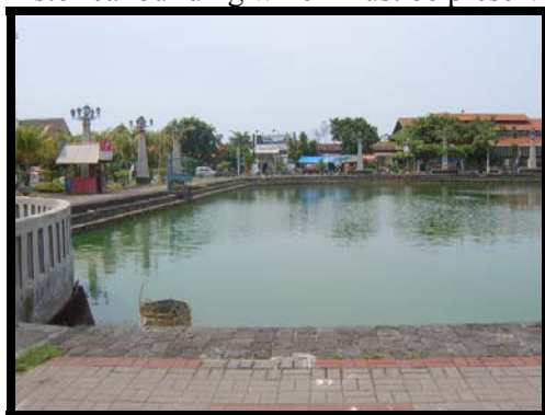
Tawang polder used as retention completed with pump
