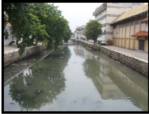
Main drainage system which cannot flow the water directly because of trash and sedimentation
