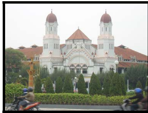
Cultural Building ( Lawang Sewu ) of Semarang City which must be preserved from flooding
