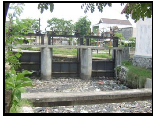
Water channel with full of trash, so the water cannot flow properly
