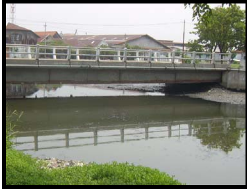
Sedimentation of Semarang River causing bridge clearance decreases annually
