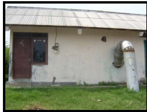
Housing pump is a facility which used for control river's water level
