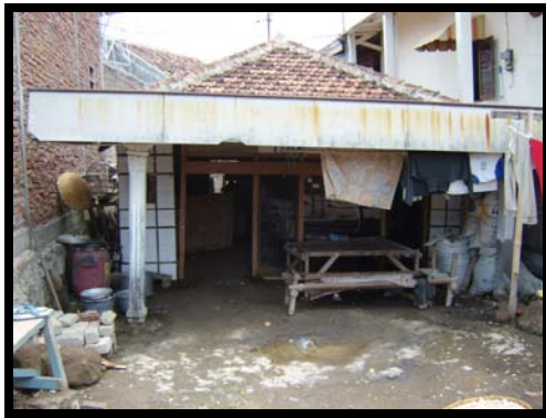
Real conditions of housing in Tanjungmas, can be seen that high of house “swallow” by land fill.
