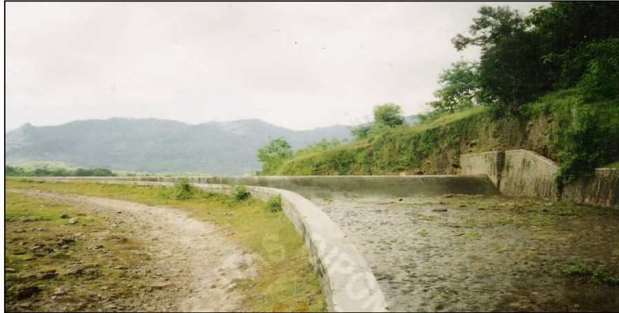
Gambar 3.3 Bangunan Pelimpah (Spillway)
