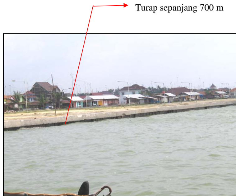
Gambar 3.2. Turap Penahan Tanah
