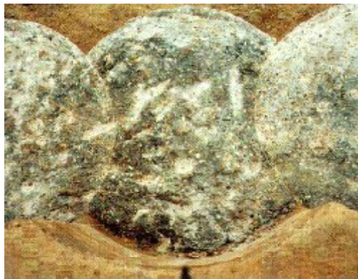
Gambar 2. 6. Dinding Penahan Tanah Bored Pile
