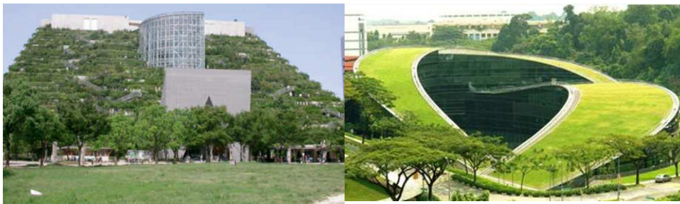
Gambar 2. – Bangunan hijau/ green building sumber : Sustainable Building Design Book , 2005.
