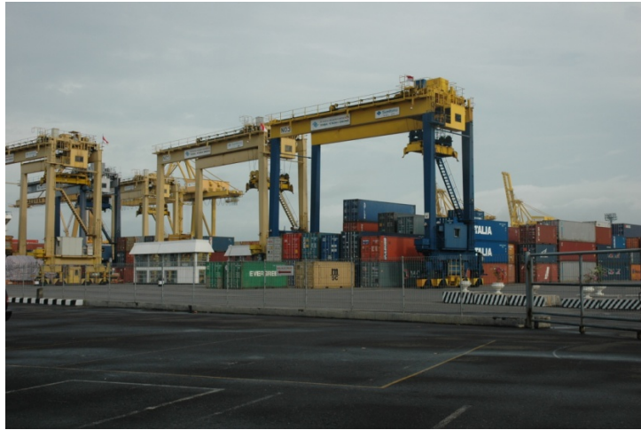
Gambar 2.5 Transtainer/RTG (Rubber Tyred Gantry)
