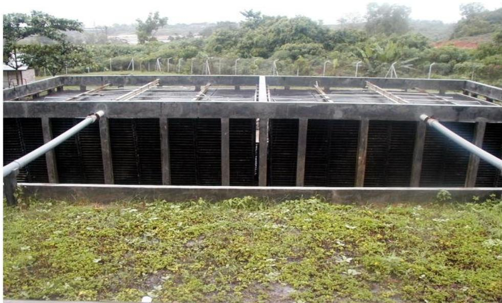
**Gambar 7. Bioreaktor/Aerator/*Trickling Filter***
